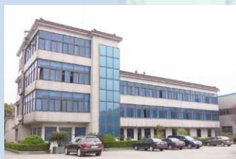
Hengye Bearing Materials Co.,Ltd (Changzhou)
